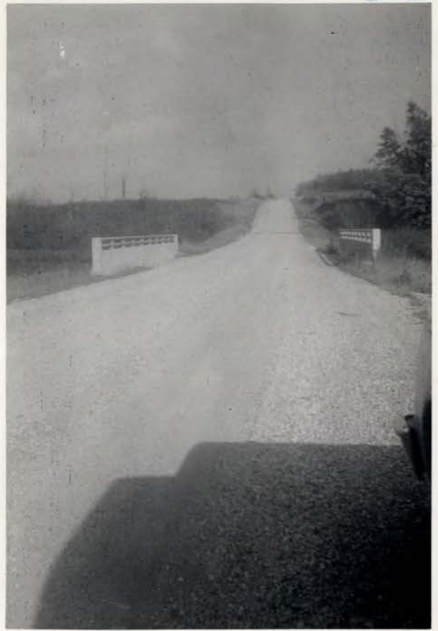
Co. Rd. 52 Bridge King Bridge 1947- Railings complid in 66-67
